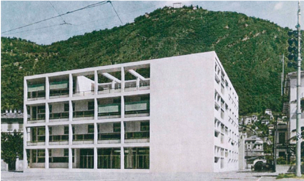
Figure 5. Old photo of the main façade on Piazza del Popolo, with the original green roller curtain system.
